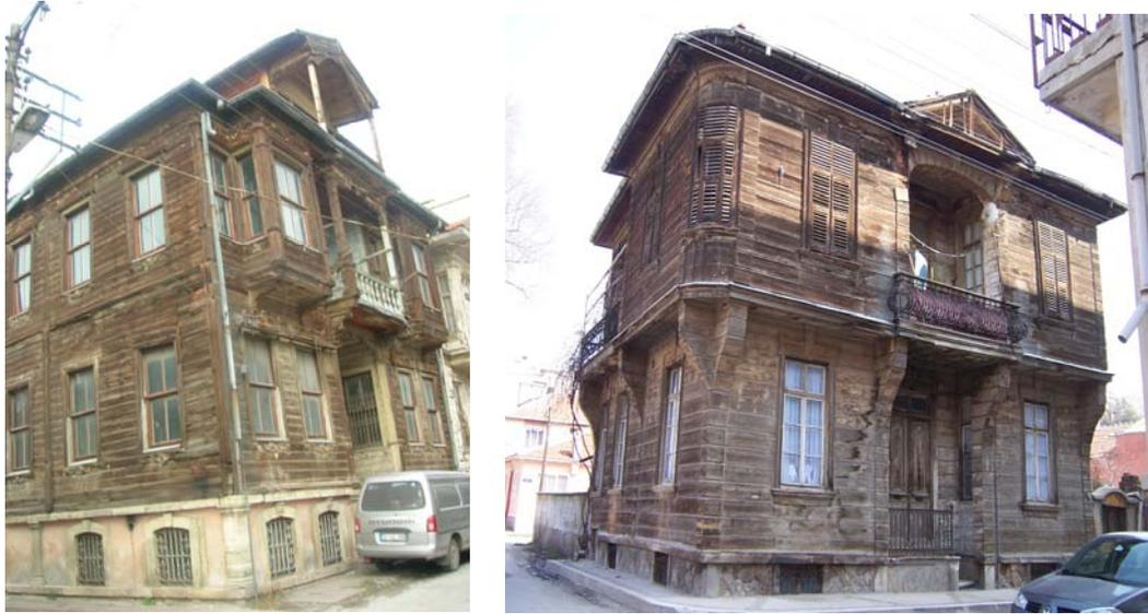
*Photo 2. Coating carcass system with timber*
