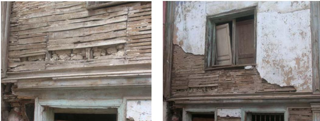
Photo 1. Coating the Wooden Carcase Buildings with Battening Coat
